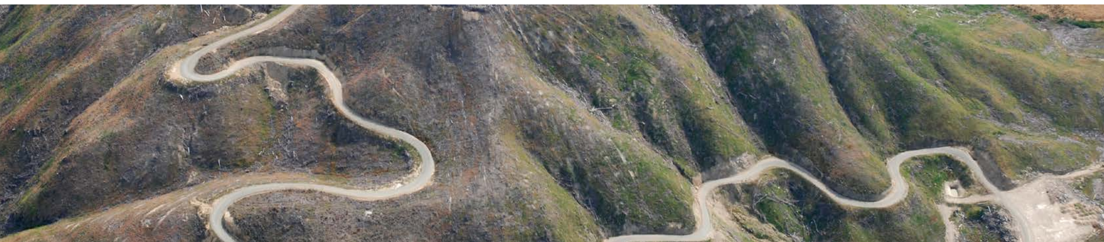
Logging of commercial pine plantations are a common sight in north Marlborough.
