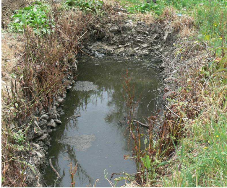
Figure 8: An example of a small milking shed effluent holding pond used for spray irrigation to land. (Bob Wilcock, NIWA).
