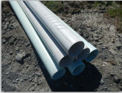
Figure 12: Gallery conduit with machine cut perforations
