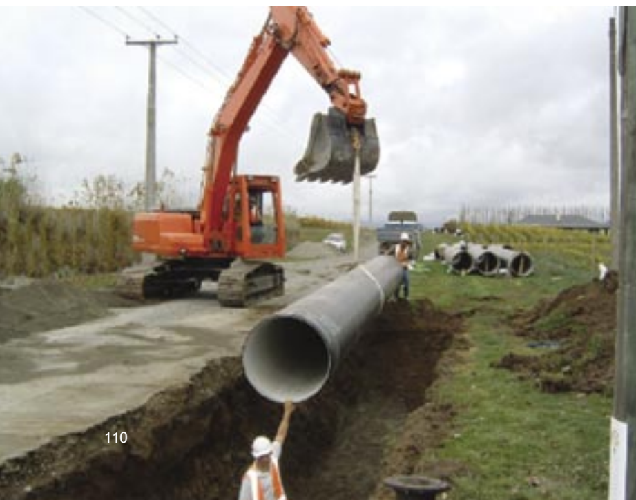
Laying of pipes for the water scheme
