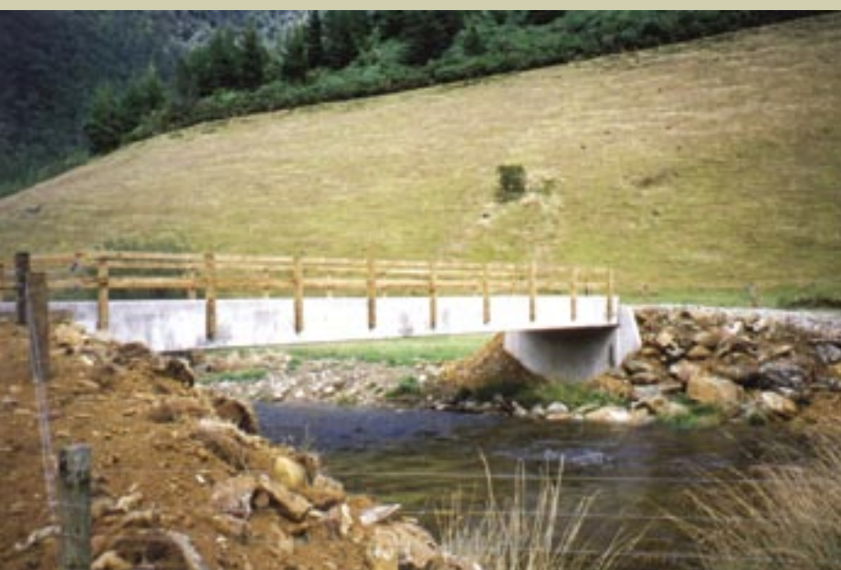
Another bridge is successfully installed, avoiding the need for dairy cows to cross directly through the river
