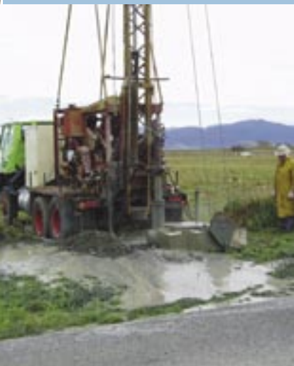
Drilling a well on the lower Wairau plain.
