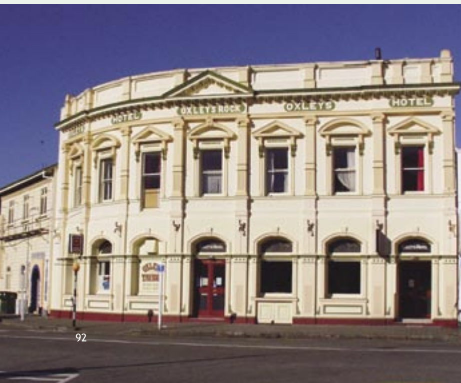
Facade of Oxleys Hotel - Picton (Class A heritage building)
