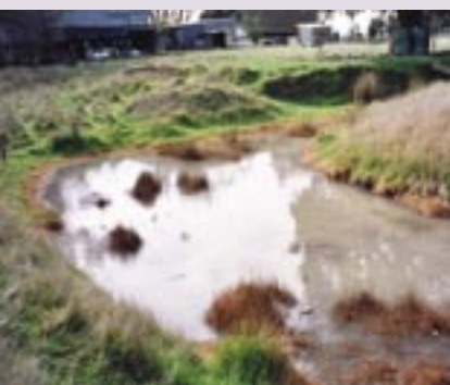
Winery effluent overflowing into waterway
