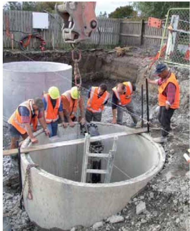
Upgrading sewerage infrastructure
