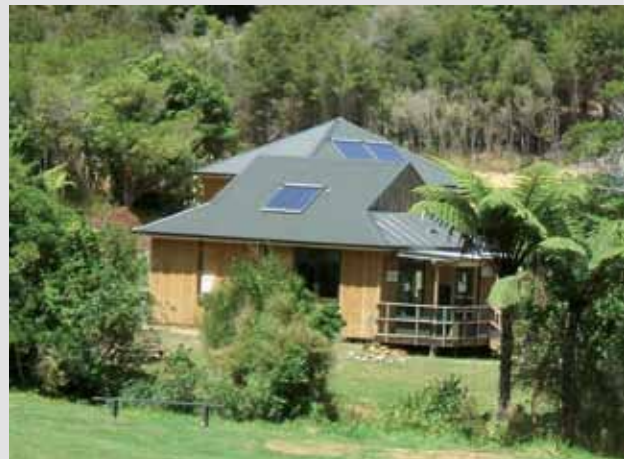
Solar panels - Mistletoe Bay Trust
