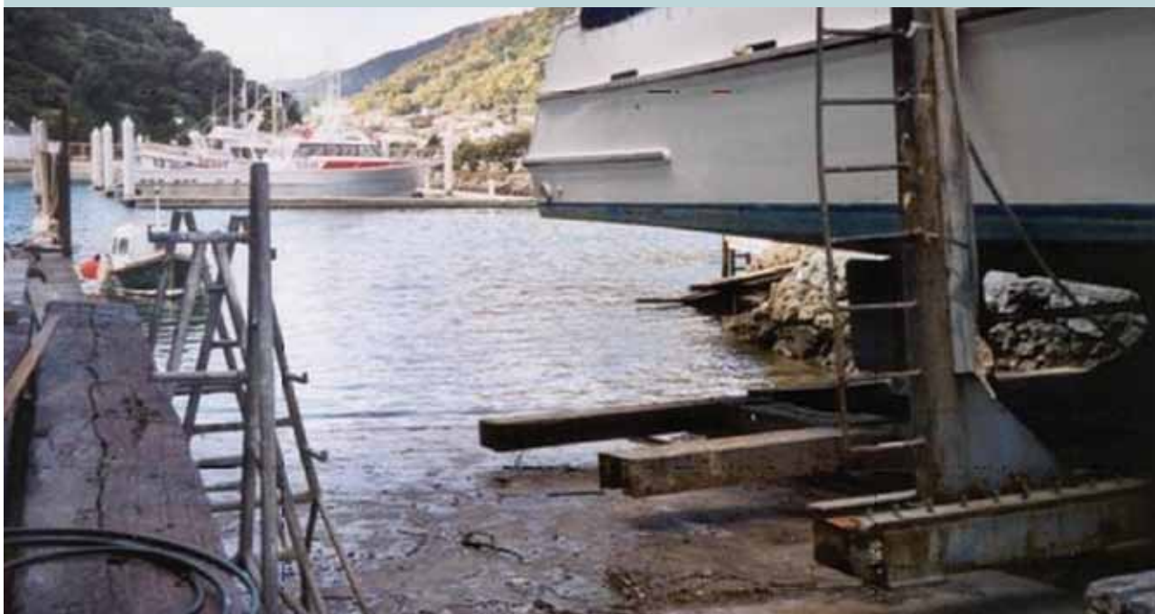
Slipway at the former Carey's Boatyard site in Picton
