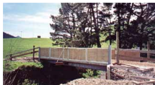
Recently installed bridge
