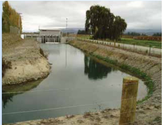
Southern Valleys Irrigation Scheme intake
