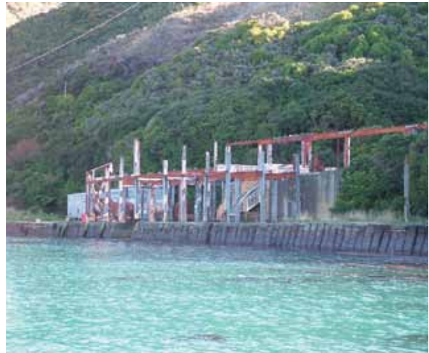
Remains of Perano Whaling Station - Tory Channel
