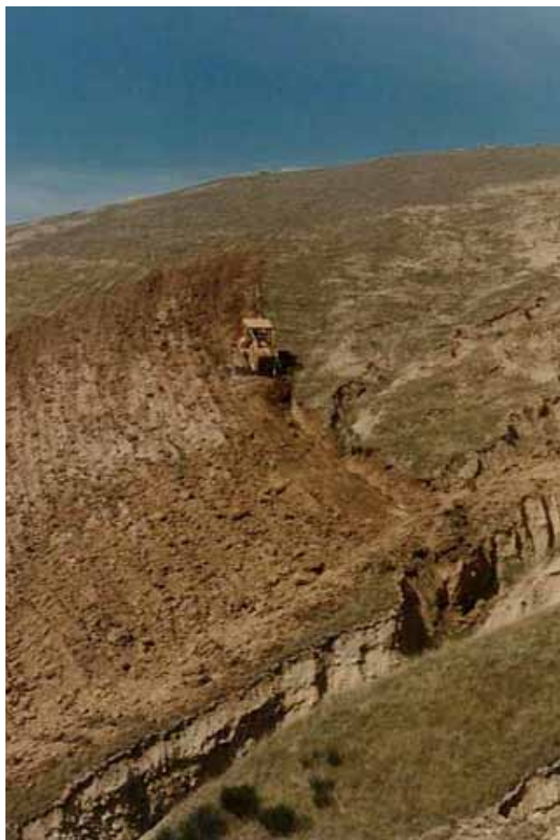
Erosion control works on the Wither Hills - 1984
