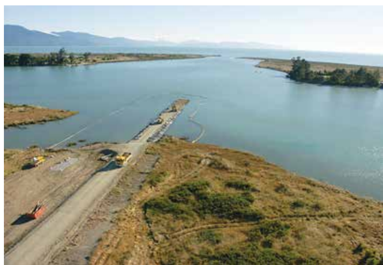
Blenheim sewerage infrastructure upgrade
