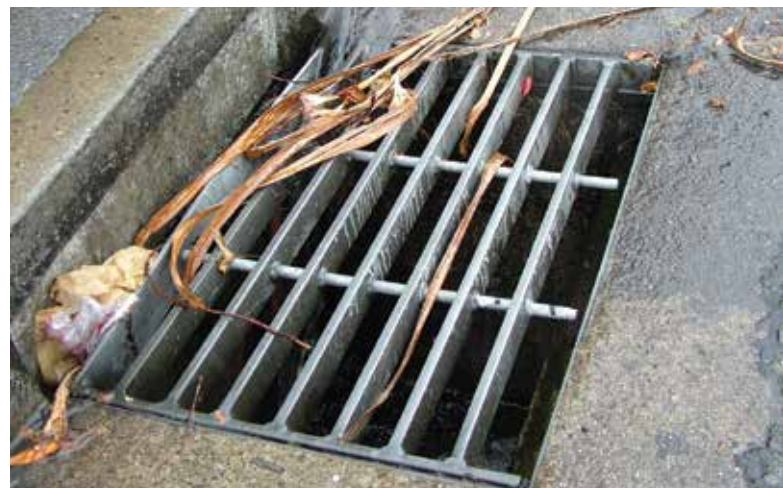
Roadside stormwater collection
