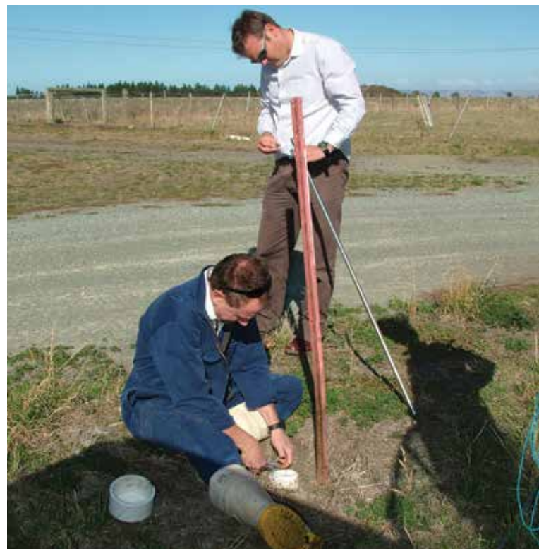
Installing groundwater recorders
