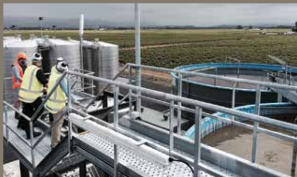
Matua Marlborough staff and Environment Awards judges discuss the reactor tanks which rely on bacteria to treat the effluent.
