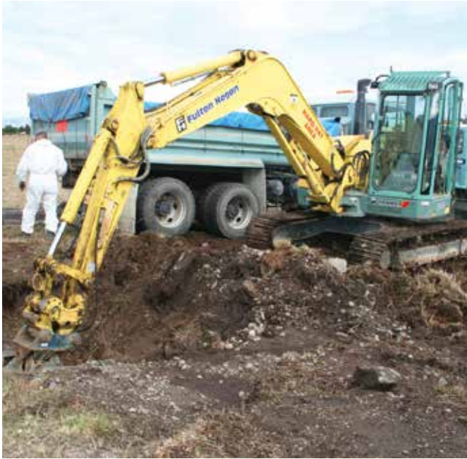
Remediation of an old sheep dip site
