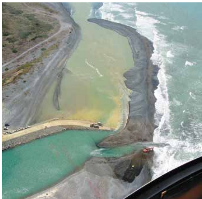
Extending the Wairau River mouth guide bank
