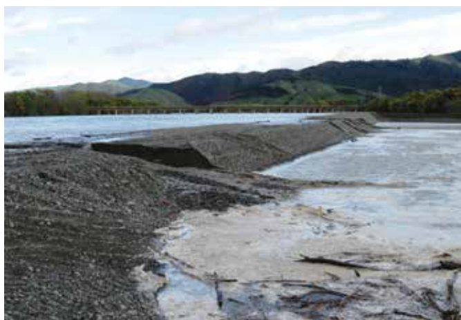
Wairau River erodible bank overtopping
