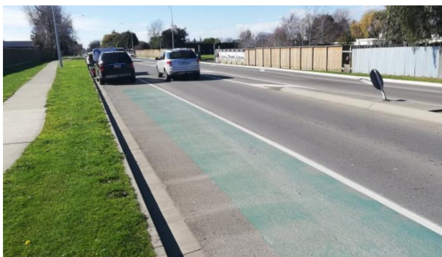
Figure 11-1: Parking in cycle lane or cycling in parking lane
