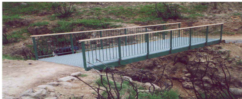
Replacement bridge within the, post Boxing Day Fire
