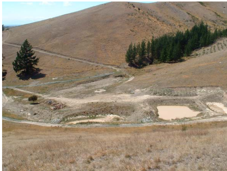
Debris Dam and Silt Traps – Mapp Stream
