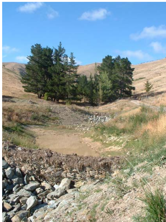
Check Dam and Rock Protection – Mapp Stream
