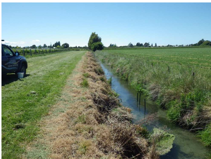
Figure 7: Kellys Drain showing the narrow, deep channel and grassy batter that has been controlled on the left bank.
