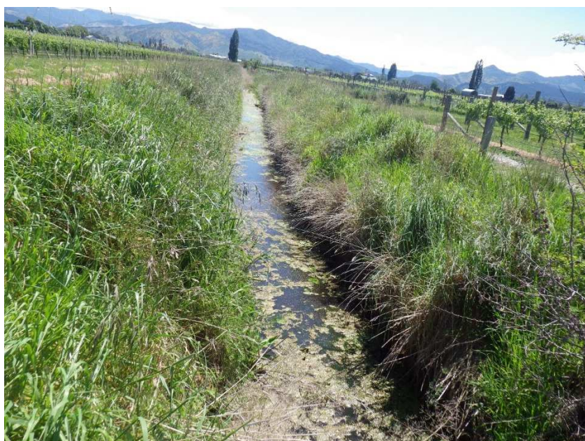
Figure 4: Drain C showing the narrow, shallow channel and grassy batter.
