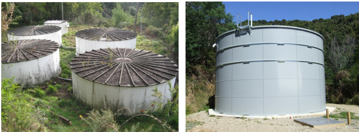
Figure 4-4 Havelock reservoirs before and after upgrade
