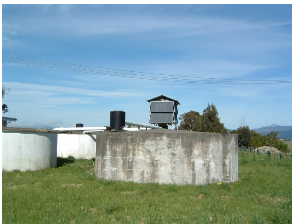
Figure 4-3 Pre-cast concrete slab and ferro-cement reservoirs at Weld Street Blenheim, The Elevation in Picton and at Renwick.
