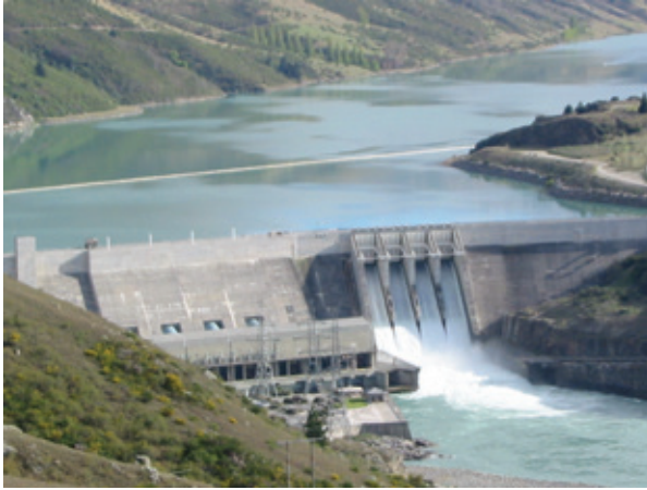
Figure 6.5: Concrete Gravity Dam – Clyde Dam (provided by Contact Energy)
