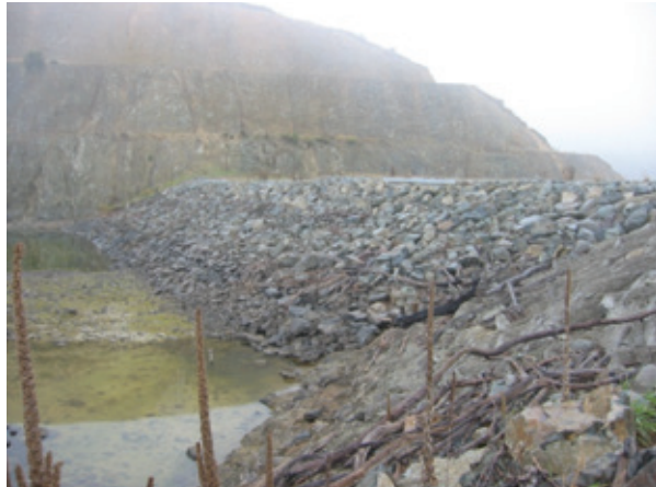
Figure 6.19: Orifice Spillway – Lower Huia Dam (provided by Watercare Services)
