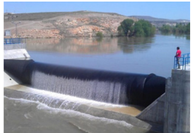
Figure 6.16: Rubber Dam
