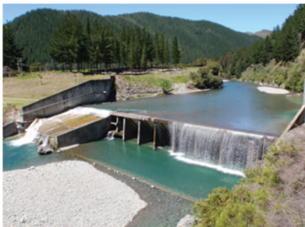
Figure 6.8: Concrete Buttress Dam – Branch Dam (provided by TrustPower)
