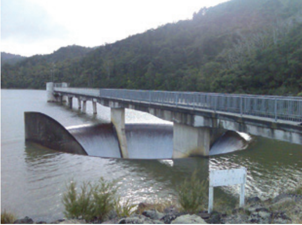
Figure 6.19: Orifice Spillway – Lower Huia Dam (provided by Watercare Services)
