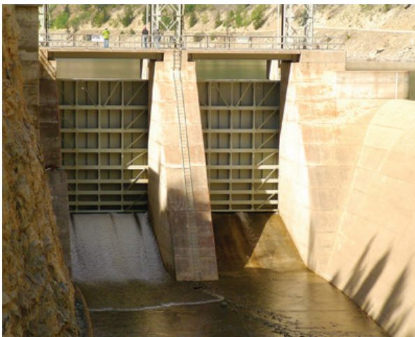
Figure 6.14: Vertical Lift Wheel Gate
