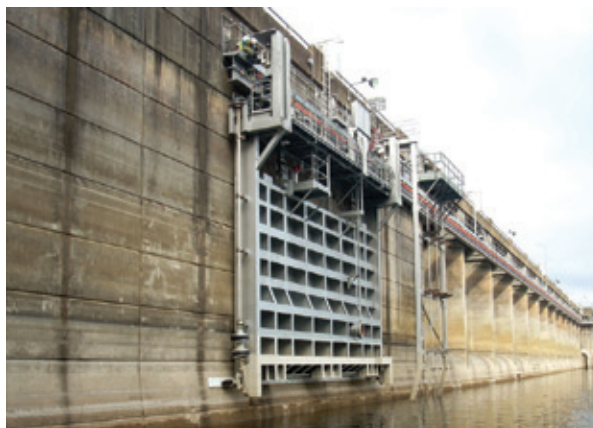
Figure 6.17: Upstream Bulkhead
