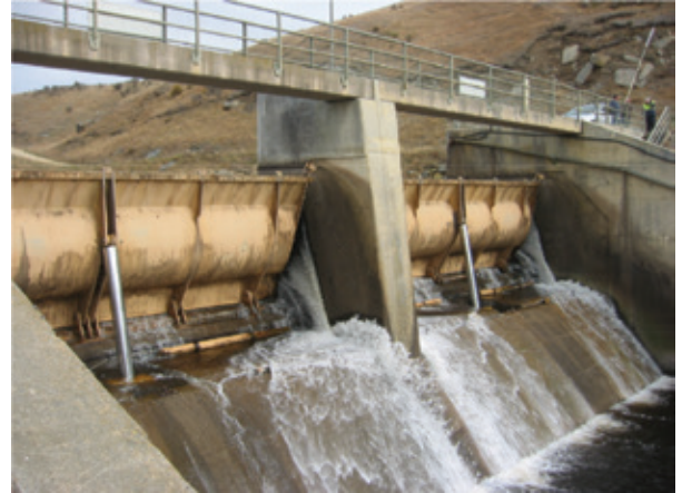
Figure 6.15: Flap Gate at Paerau Weir (provided by TrustPower)
