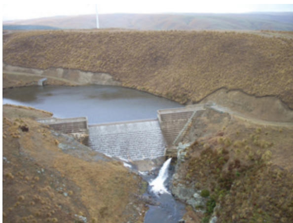
Figure 6.6: RCC Dam – Horseshoe Bend Dam (provided by Pioneer Generation)
