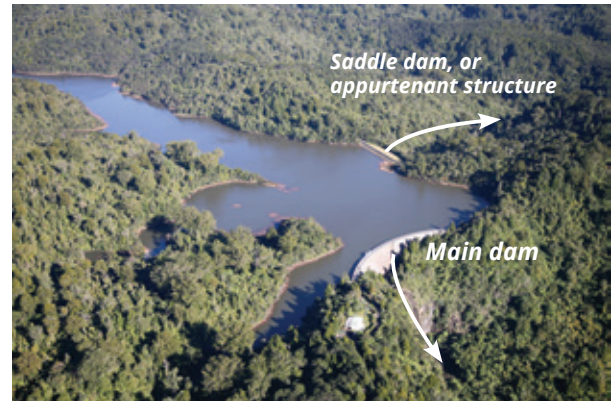
Figure 4.1: Example of Main and Subsidiary Dams or Appurtenant Structures (e.g. gated spillway) with Different Features and Dam-Break Flow Paths (provided by Watercare Services).
