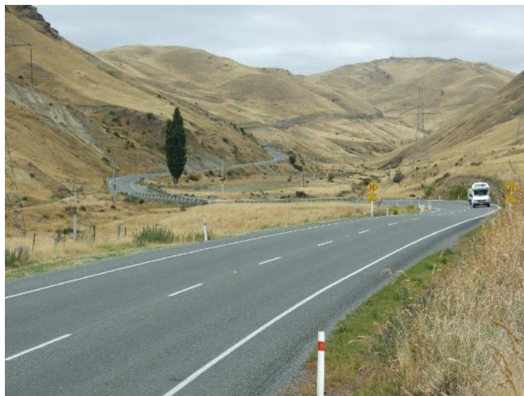
Puka Puka Weld Pass SH1, Marlborough
