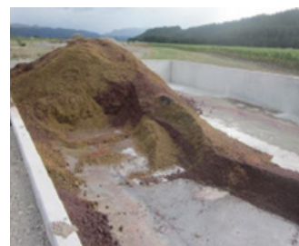
Sealed storage area with leachate collection
