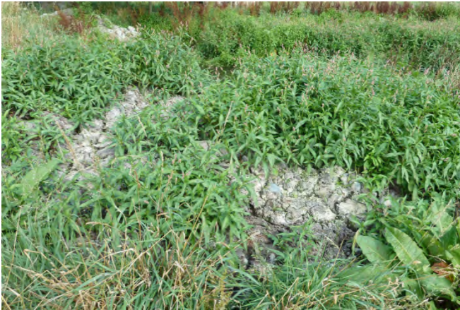
Effluent pond is full with vegetation and solids build-up
