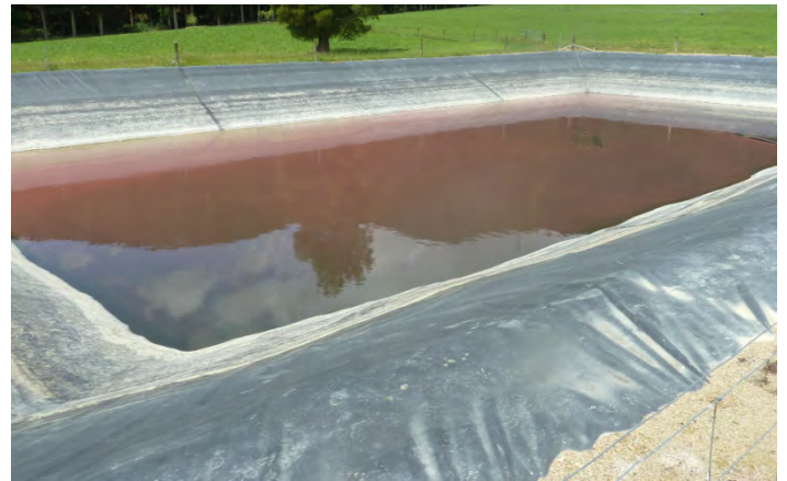
Effluent pond has plenty of free-board available
