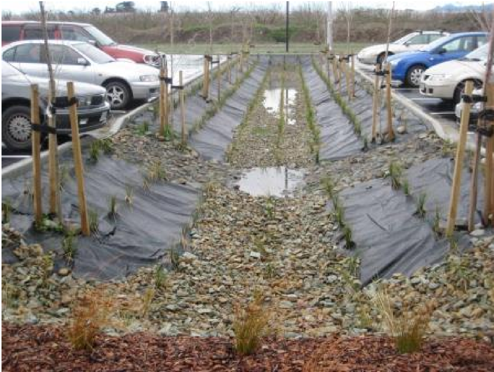
Storage Area – 9 August 2012
