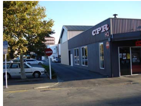
ABOVE FIG. 5-22: Poor quality pavement and insufficient width of the footpath in Wynen Street.
