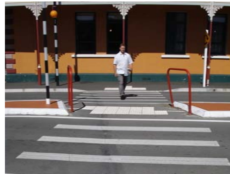
ABOVE FIG. 5-18: The column on the end of the crossing (behind the gentleman on the photo) could pose a safety hazard for the elderly and the disabled
