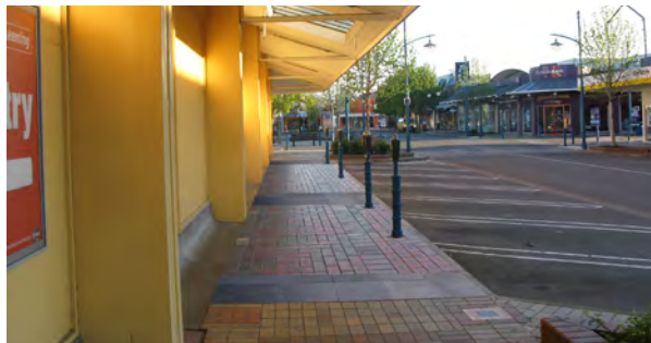
Photoshop illustration of retrofitting cut stone and clay paving into existing asphalt
