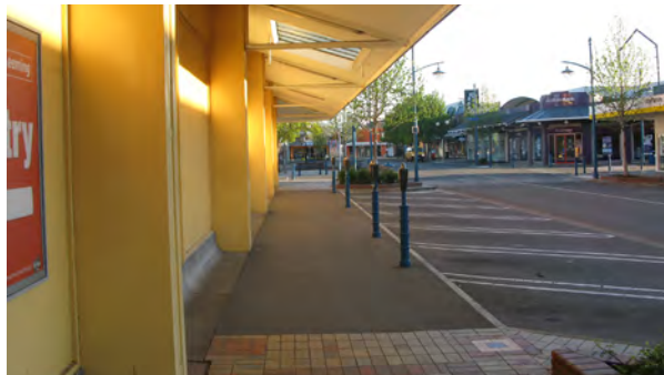
Existing clay paving and asphalt
