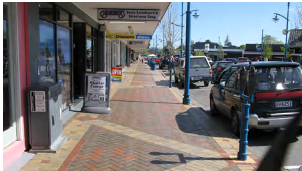
Existing paving - clay paving
