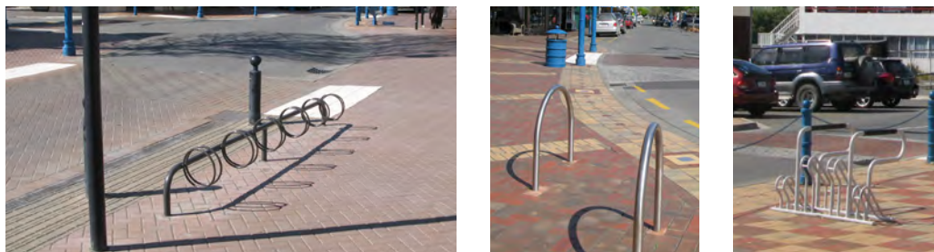
Three main types of existing cycle racks within the considered area
