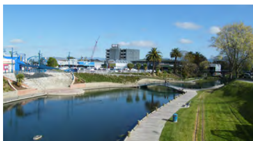
View of the site from S.H.1 bridge
