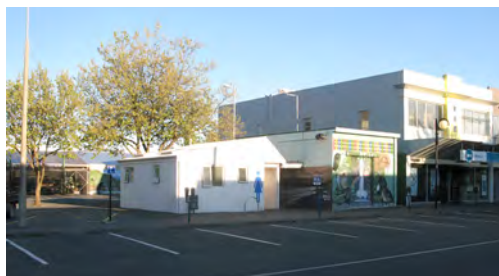
Existing toilet block and substation
