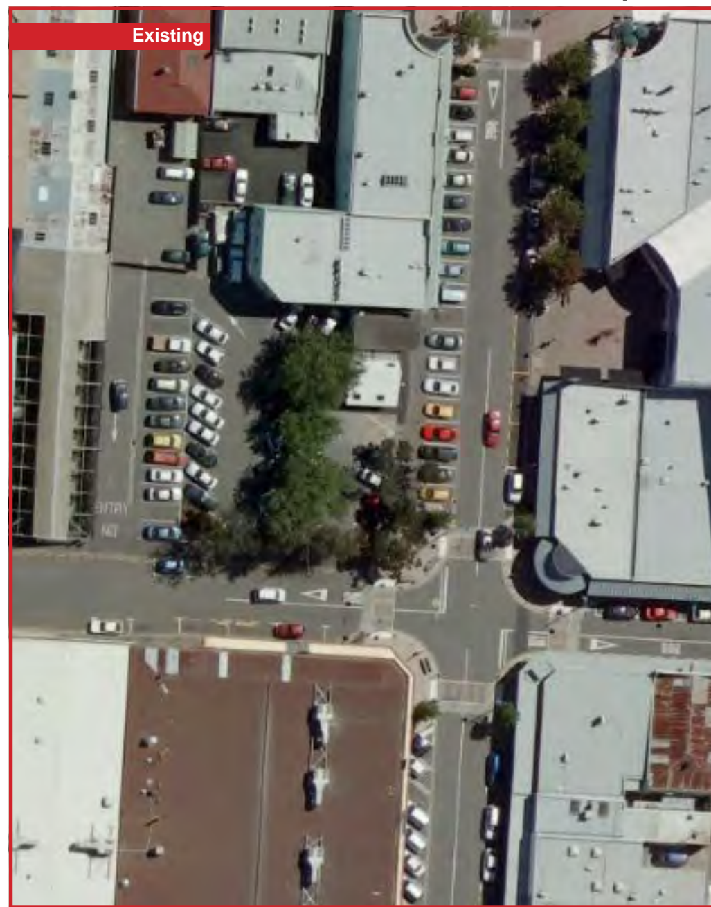
Fig. 35: Aerial photo of existing Queen Street Car Park
