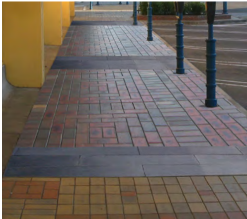
Photoshop illustration of retrofitting cut stone and clay paving into existing asphalt
