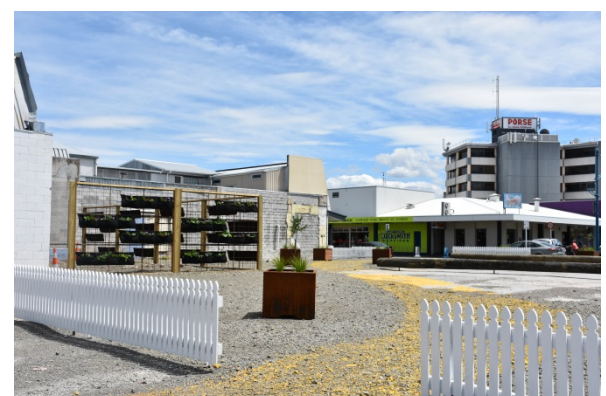
Figure 11: Pocket park that has been created on demolished building site on High Street.
