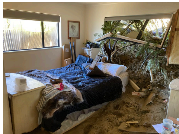
DS3 – Moderate: Repairable structural damage.
