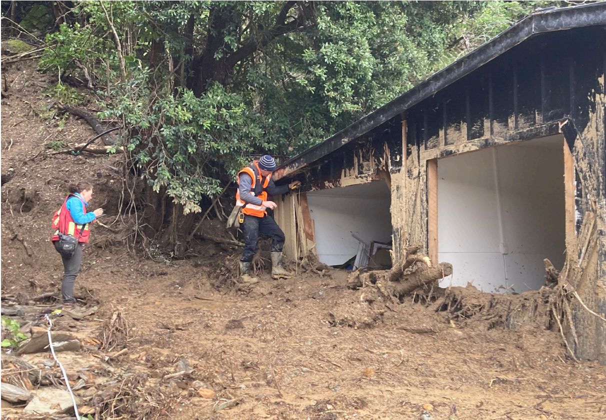
Figure 2.5 Surveying of landslide debris; measuring inundation along building side. We measured maximum run-up signs (here, above the building windows) not the height of the debris at the time of survey (here, at the base of the windows).
