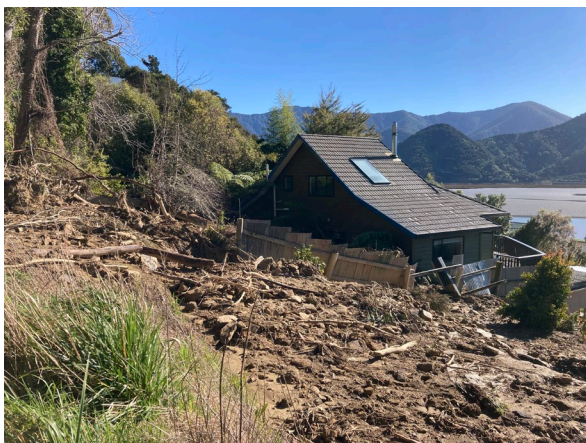
DS3 – Moderate: Repairable structural damage.
