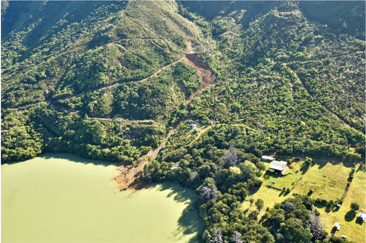
Figure A1.3 Debris slide/slump and flow initiated from older forestry landing, Pelorus Sound, near Black Point.
