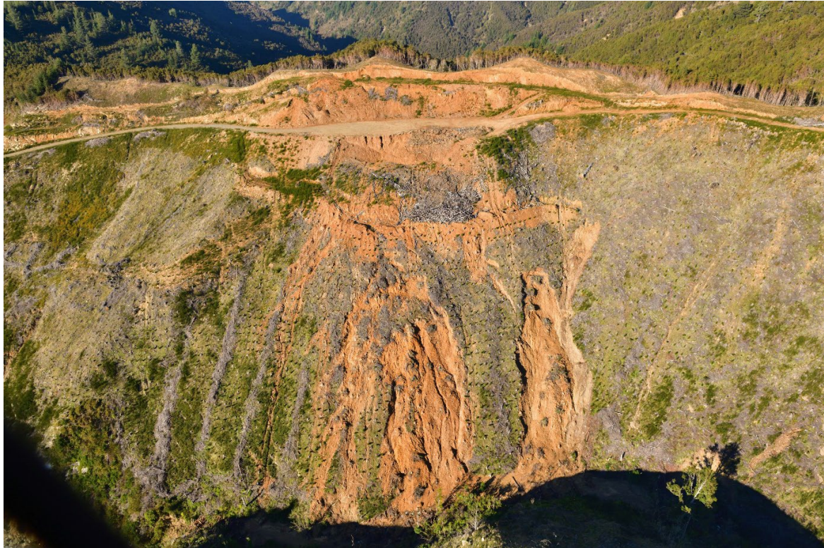
Figure A1.7 Mid-slope failures and debris avalanches/flows on newly planted exotic forest slope. Also possibly shows a collapsed landing or skid site. Root raking has occurred up and down the slope, which means that a machine has been down the slope and the surface was likely very disturbed prior to failure.
