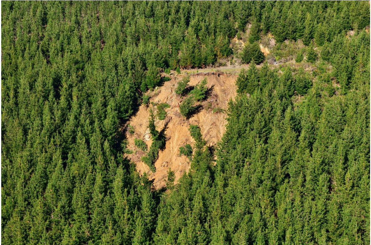
Figure A1.9 Debris avalanche from a collapsed older landing, constructed from slash and fill, in exotic forestry near Havelock.
