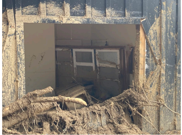
DS4 – Severe: Irreparable structural damage.
