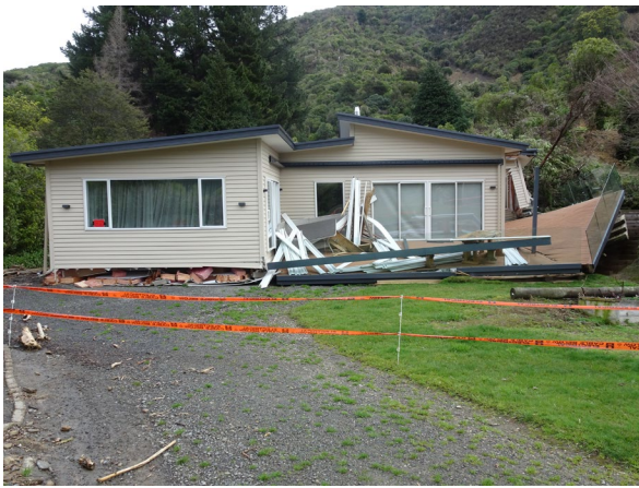
DS5 – Critical: Structural integrity fails.
