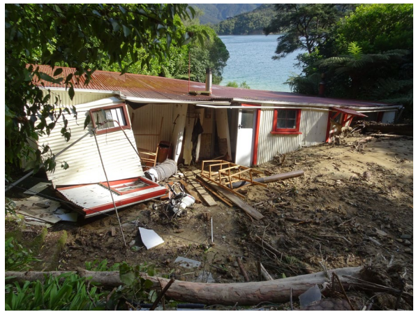
DS5 – Critical: Structural integrity fails.
