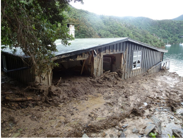
DS4 – Severe: Irreparable structural damage.
