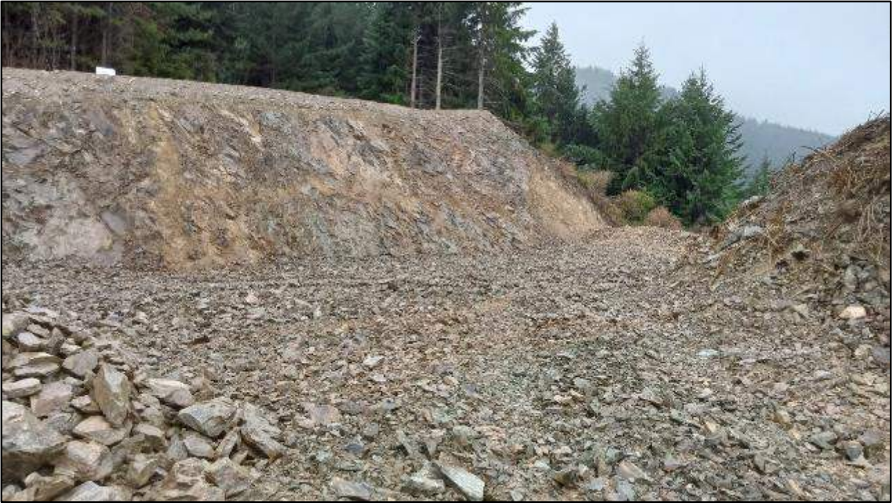
Figure 9 – top bench forming
