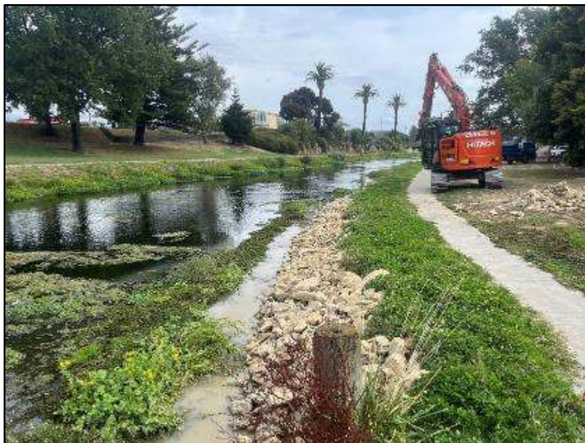
Figure 4 - 13t digger placing riprap rock at Taylor River
