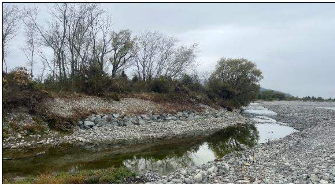
Figure 1 - 350t Rockwall at top end of existing riprap structure
