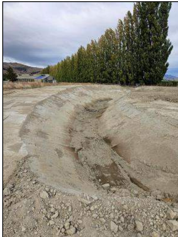
Figure 7 – realigned section of Town Branch Drain
