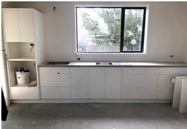
Fig. 9 – Senior Housing development, Kitchen install
