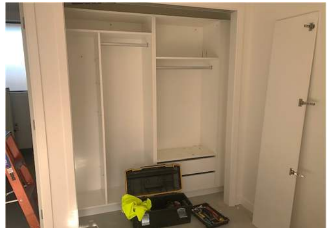
Fig. 10 – Senior Housing development, Wardrobe install
