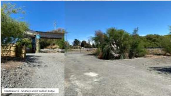
Road Reserve - Southern end of Section Bridge
