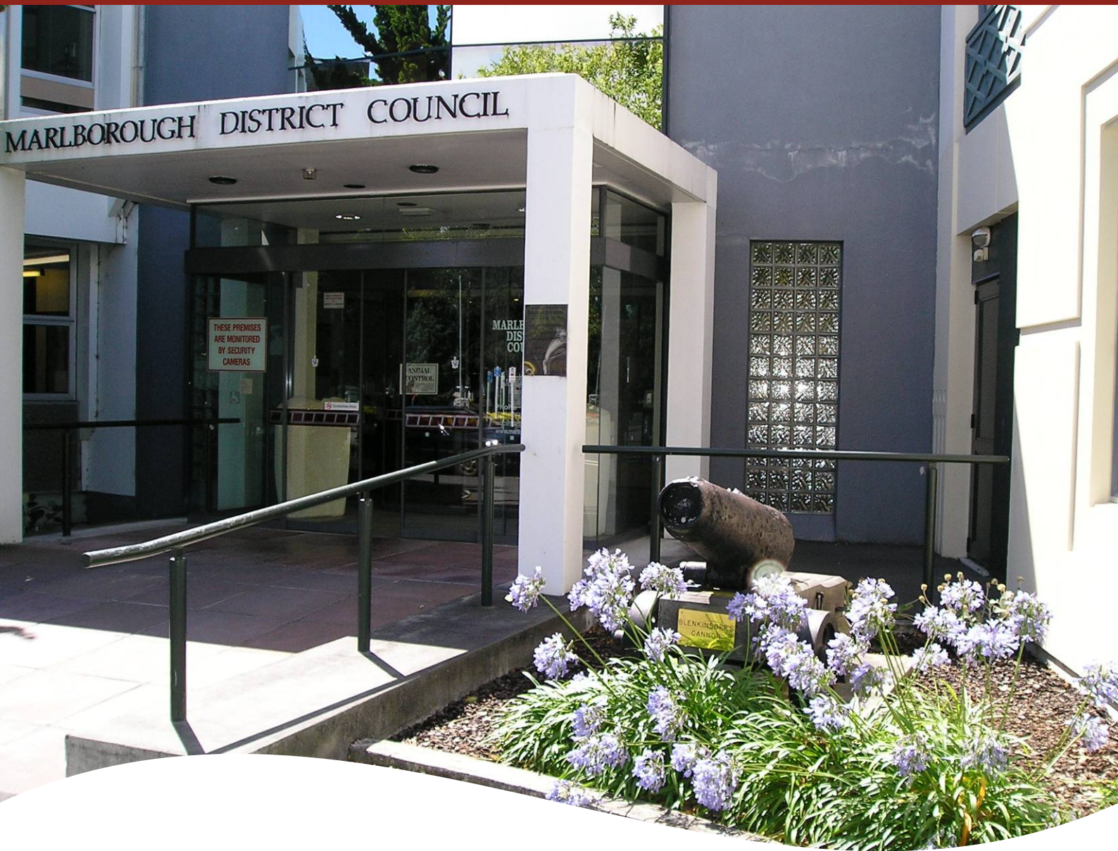
Picture: Marlborough District Council Building, Blenheim
