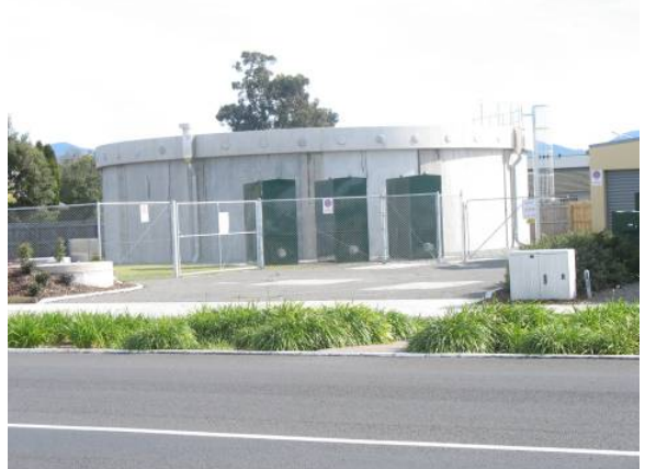
Middle Renwick Road Water Treatment Plant
