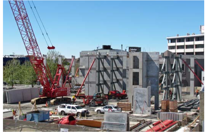
Commencement of the new carpark building, Alfred Street, Blenheim
