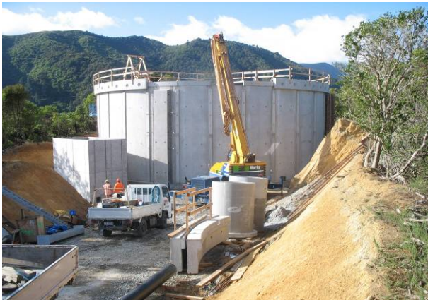
Construction of the Victoria Domain Reservoir, Picton
