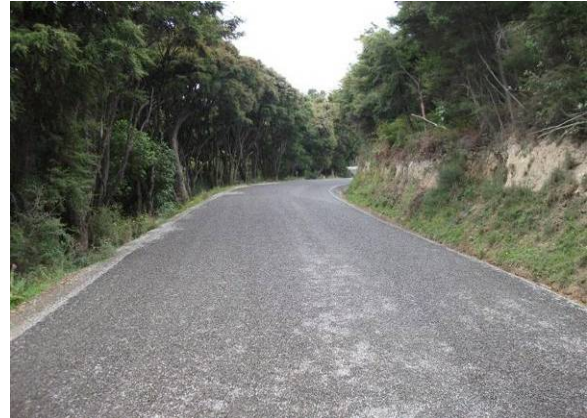
Figure 1: Kenepuru seal extension after construction
