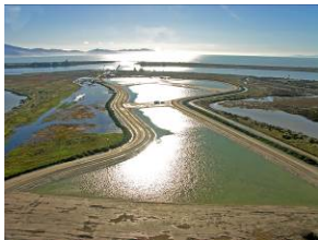
Sewerage upgrade – new wetlands
